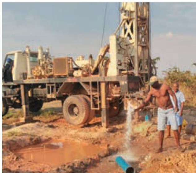
Water-well drilling in Angola (above and below)
