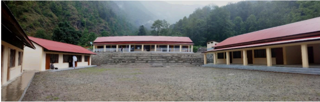
Relocated school in Golmadevi 2019 © Daniel Schwitter
