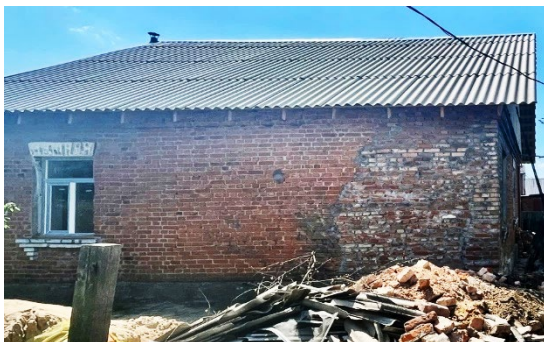
Village house repaired with used bricks (Image D. Wyss)
