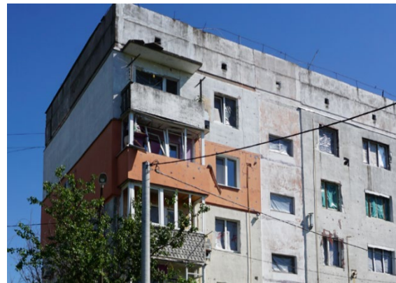
A Khrushchevka-apartment in Makariv with an external thermal insulation added by the homeowner (Image Daniel Wyss)
