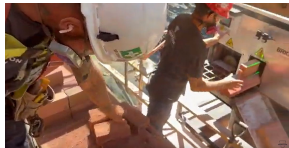
In-Situ brick trimming in Canada Image: Youtube
