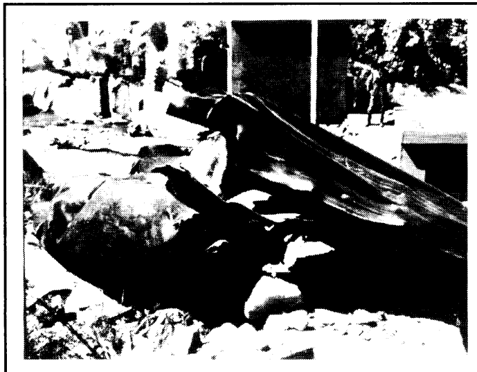
Figure 34: Destroyed penstock due to water-hammer Photo by: W. Roth
