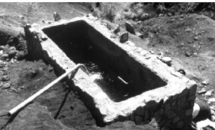
7. The last construction part of the building is to cover the tank. Therefore, the precast slabs are put in place. One special designed cover with an opening for a tank with a manhole (for maintenance reasons) is put a the side where the supply washout and overflow installations are.
