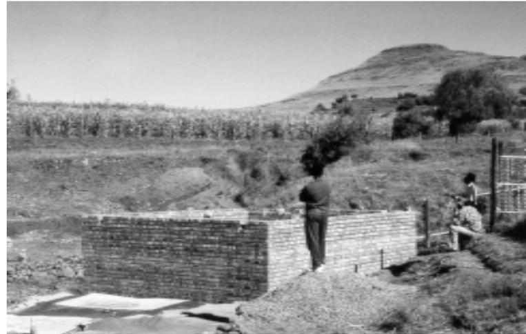
makes cement block masonry very economical. For cement blocks the stretcher bonding is most commonly used.
