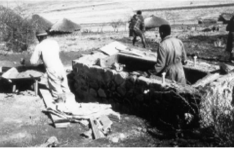
5. During the time of plastering the pointing of the outside wall can be done.
