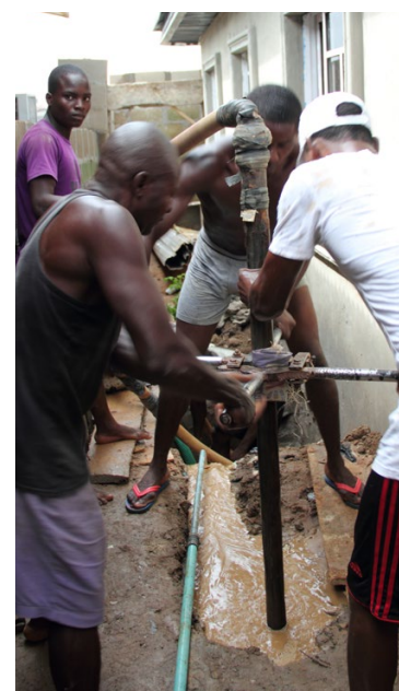
Drilling for household supply in Lagos
