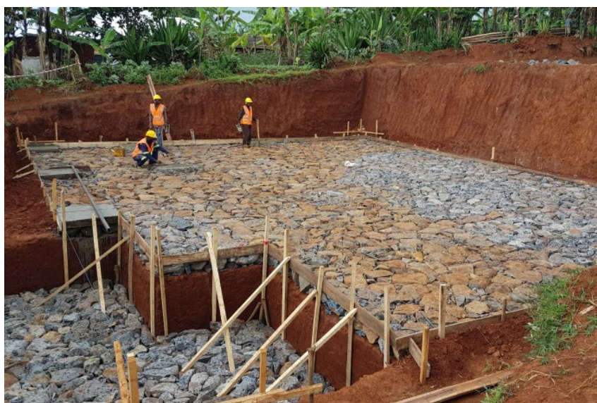
Rock fill of one of the reservoirs for the Panzi water supply systems (Bukavu town, DRC)
