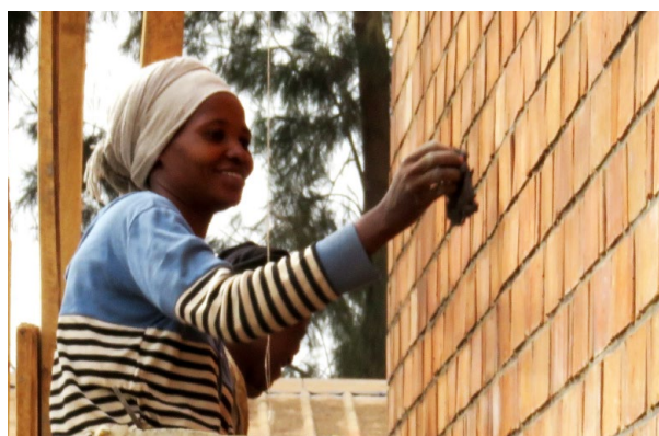
Female construction professional in charge of pointing and finishing of the "smart & green brick walls" of the Swiss Cube building at EXPO 2017. (photo: Daniel Wyss)
