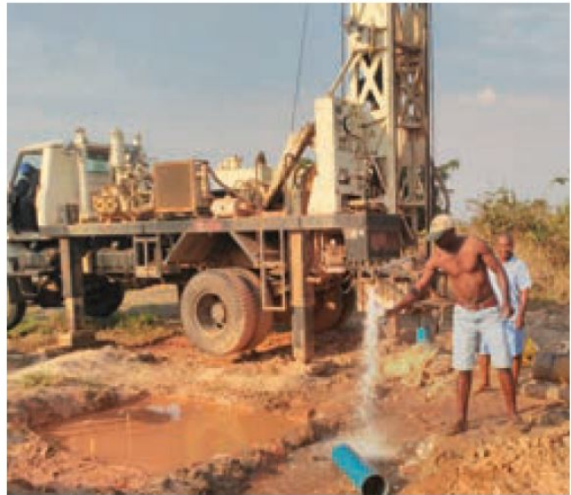
Water-well drilling in Angola (above and below)
