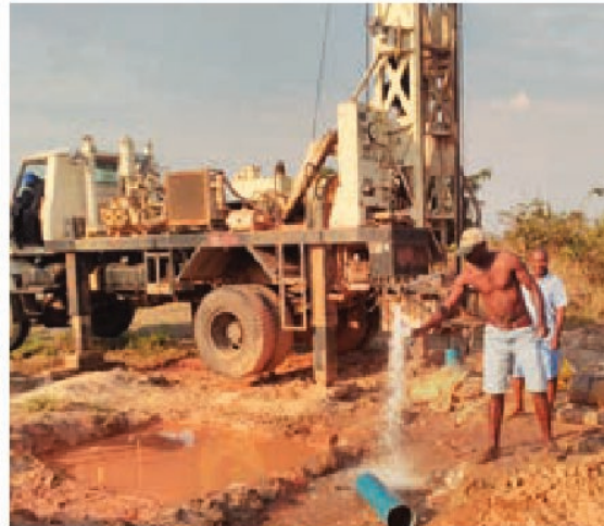
Water-well drilling in Angola (above and below)
