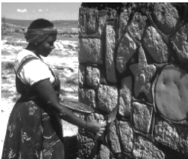
Pointing can be carried out as the construction of the blockwork proceeds, using ordinary mortar in which the blocks are bedded. This type of pointing is called struck jointing and is much cheaper than the pointing methods described below. Another method is to finish the masonry work first and then to make the pointing work with a 1:2 cement mor-
