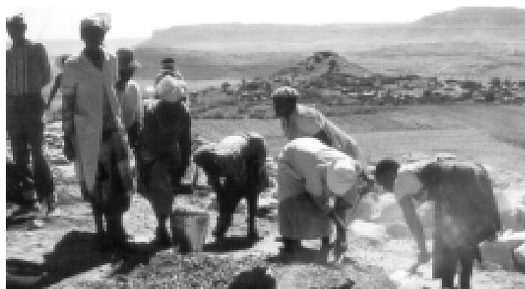
Hand mixing does not require much equipment, but a lot of man power. A batch to be hand mixed should not be larger than about 0.5 m<sup>3</sup>. Concrete should never be mixed on soil because of the proved danger of contamination by organic matters. A levelled platform has to be prepared to prevent water or fluid material from flowing out of the mixture.
