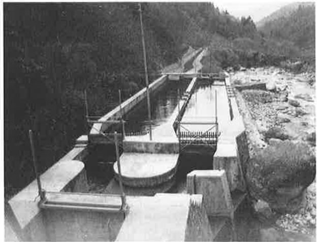
Photo 4b ... and Operation of the Sandtrap
