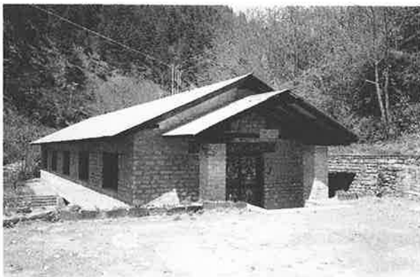
Photo 2 The Power House...
