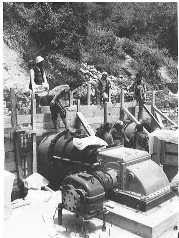
Photo 6 Construction and Installation of a Turbine...
