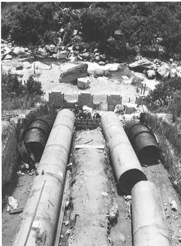
Photo 5 Construction of Twin Penstock
