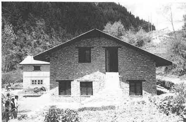
Photo 3 ... and the store cum workshop of the power plant.
