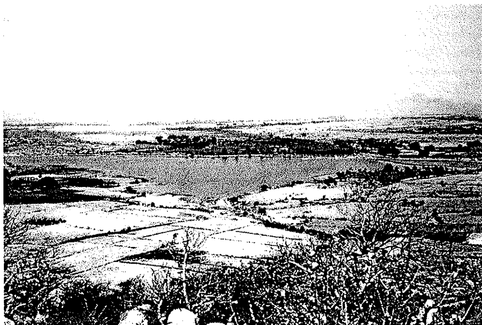
Figure 2 (photo of the tank and the surroundings at CR Palli, after heavy rainfall)
