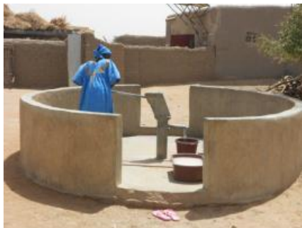
Rehabilitated and protected water source
