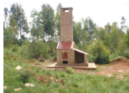
Incinerator for solid waste
