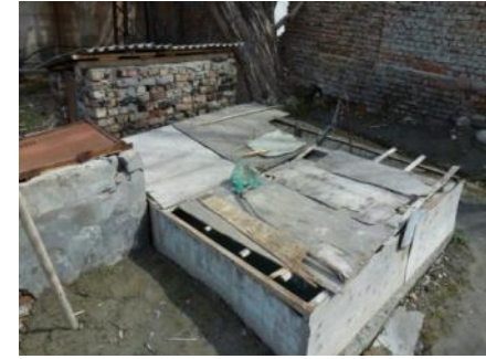
Fresh water treatment with chlorine
